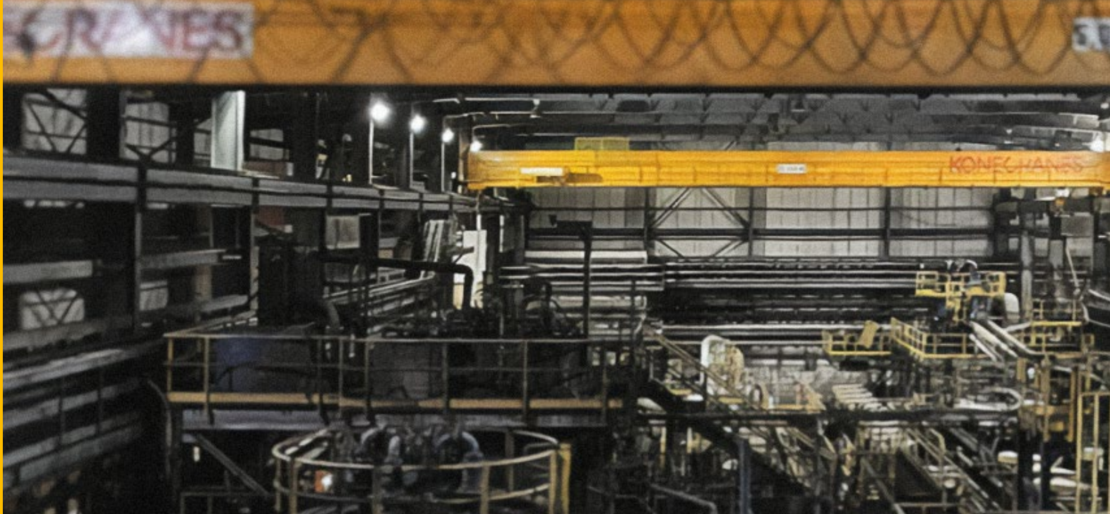
Facility cranes shown above.
